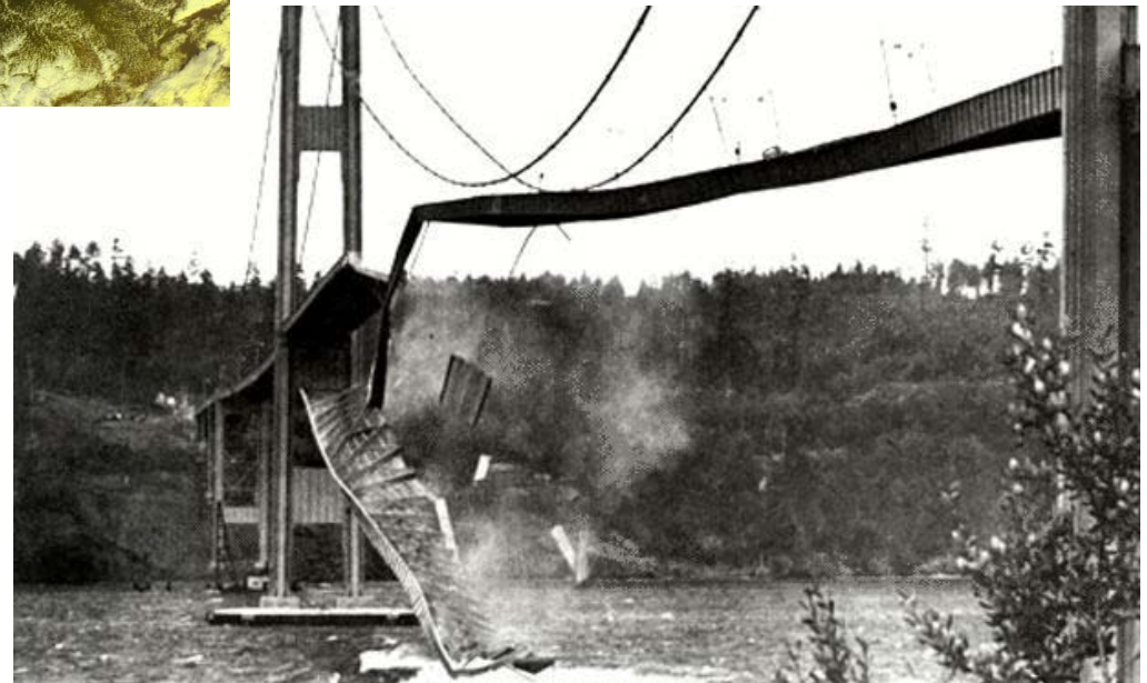
Tacoma narrows bridgeの崩壊
